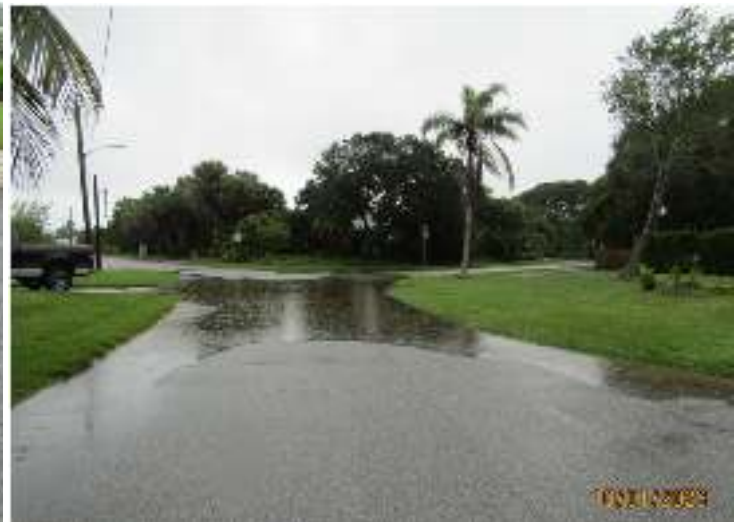
Shannon Intersecting Poinsettia/Magnolia – The water then Flows to Harland and Poinsettia. Harland has a large swale from previous stormwater work. That captures that water preventing yard flooding there. Poinsettia has no functioning stormwater underground piping. It is over 50 years old corrugated pipe. We have attempted to use the ditch witch and clean the pipe to no avail.
